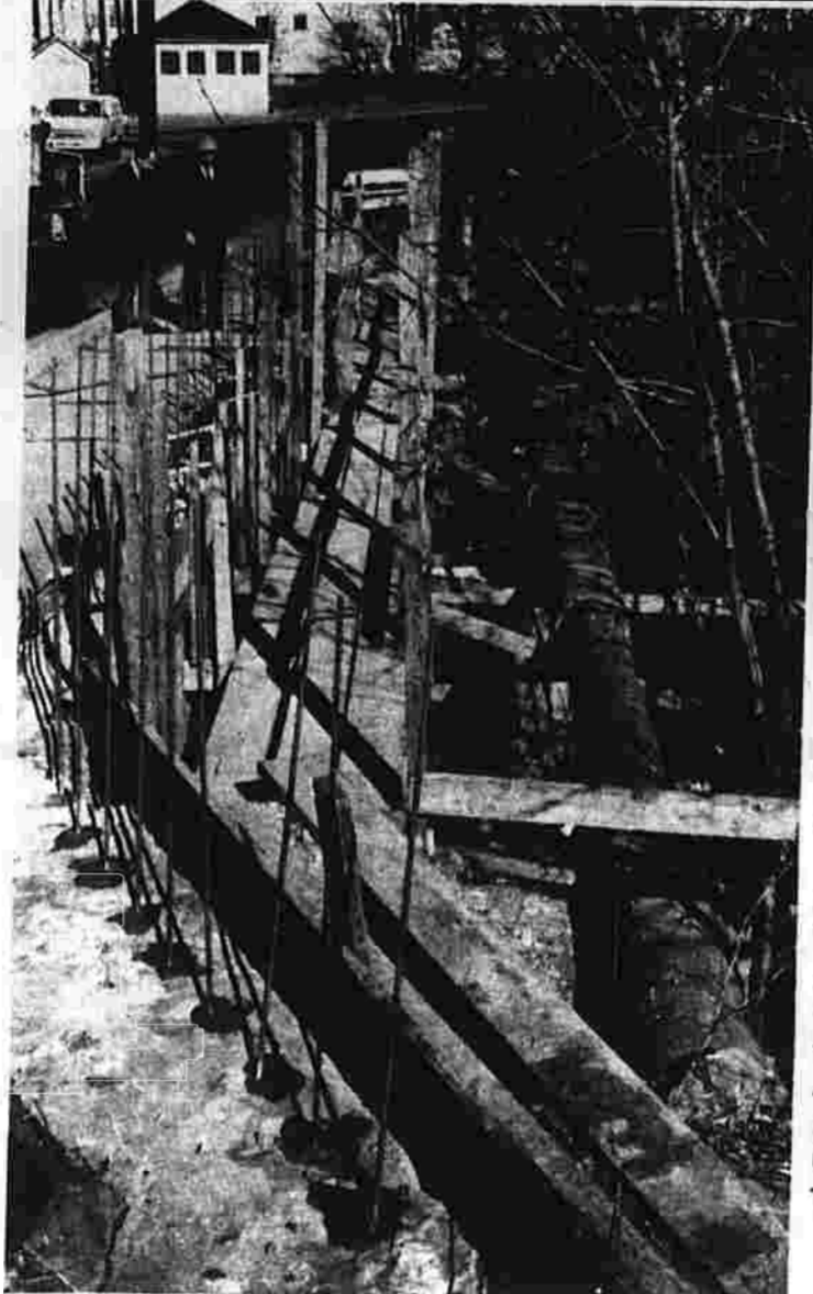
Bridge Being Repaired
